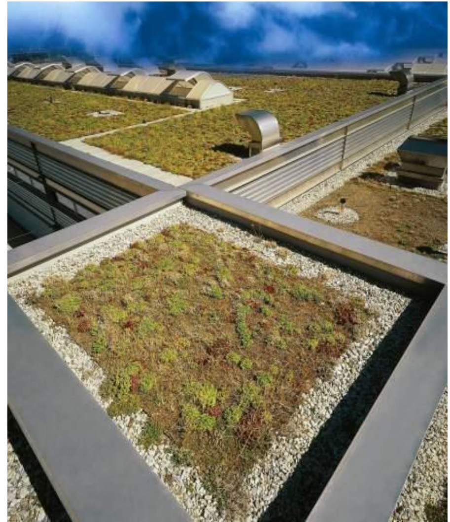
Furka-Oberalp Rail Depot, Brig, Switzerland
