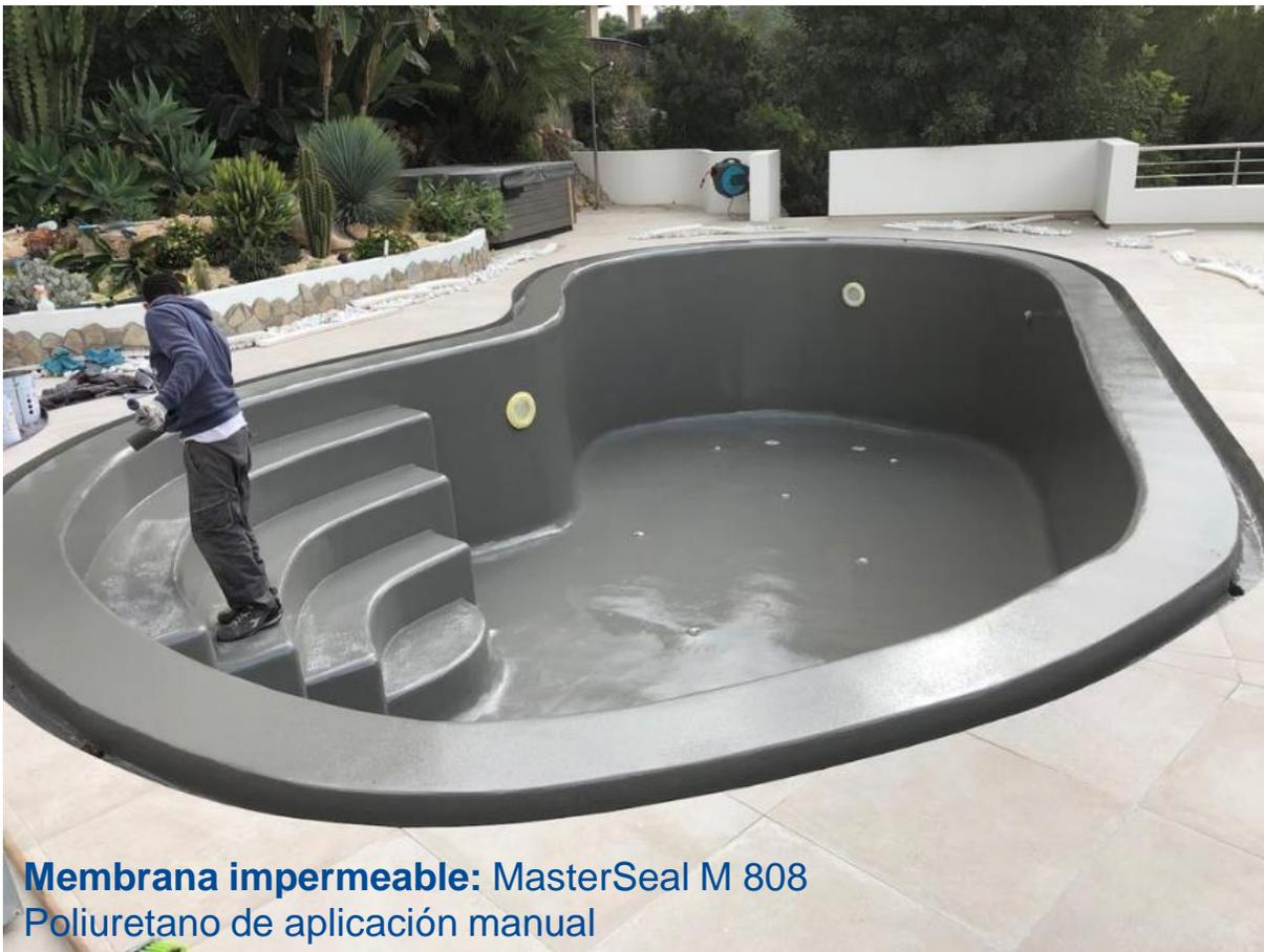
**Membrana impermeable:** MasterSeal M 808
